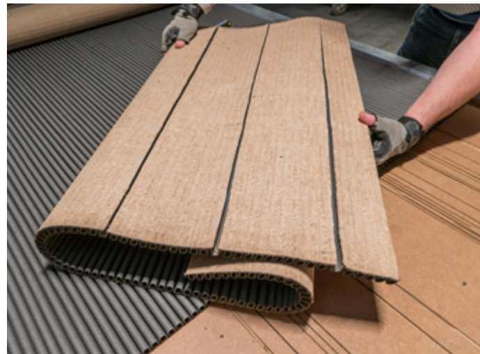
Step 2: Add relief cuts at required intervals.
