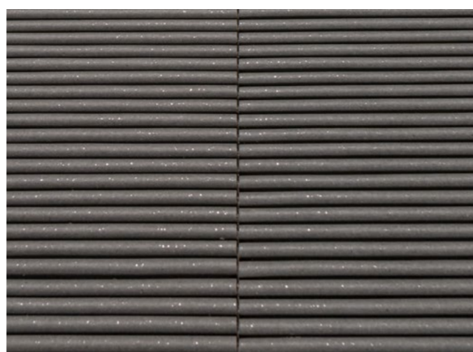
After: Ribs aligned.
